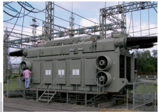
200 MVA Transformator
