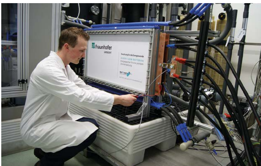
Figure 13: Redox flow battery
