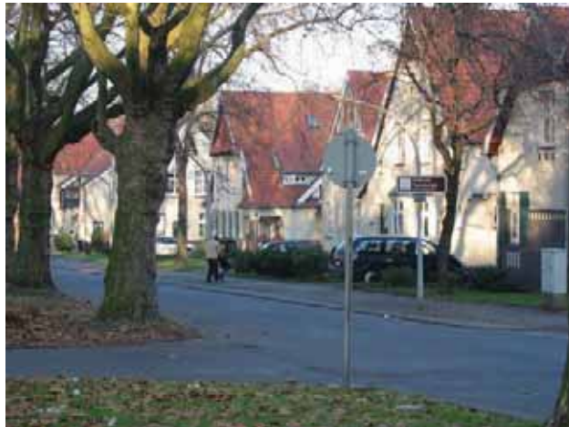
510 renovated former miner houses of the housing estate Teutoburgia will be supplied with environmentally friendly produced heat.
