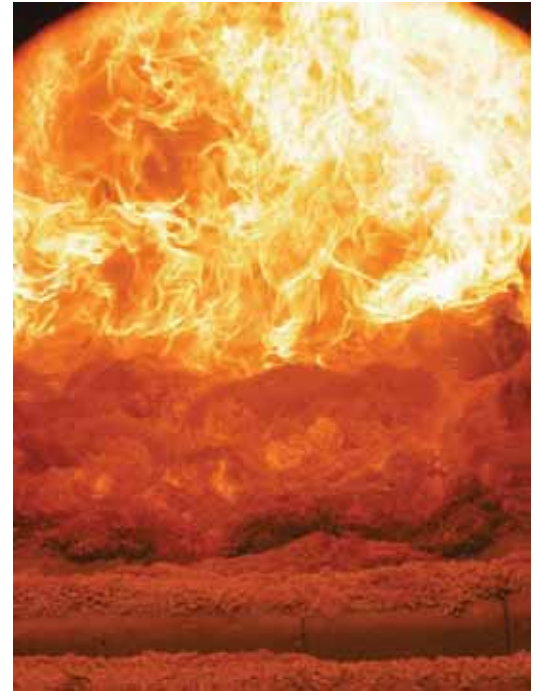
View into the combustion chamber with the help of the Hytim® Camera
